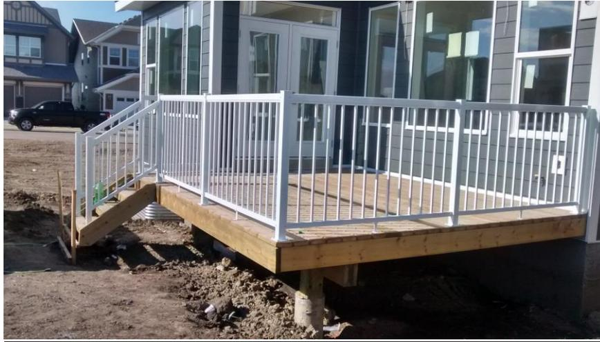
1. For decks make sure to install “key posts” “Key posts” are posts that start and end a run of rail “Key posts” are EP and CP
